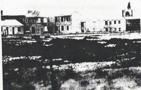
Mock village on the Dungeness peninsula in Kent which was constructed for realistic military training in Northern Ireland and urban areas.
